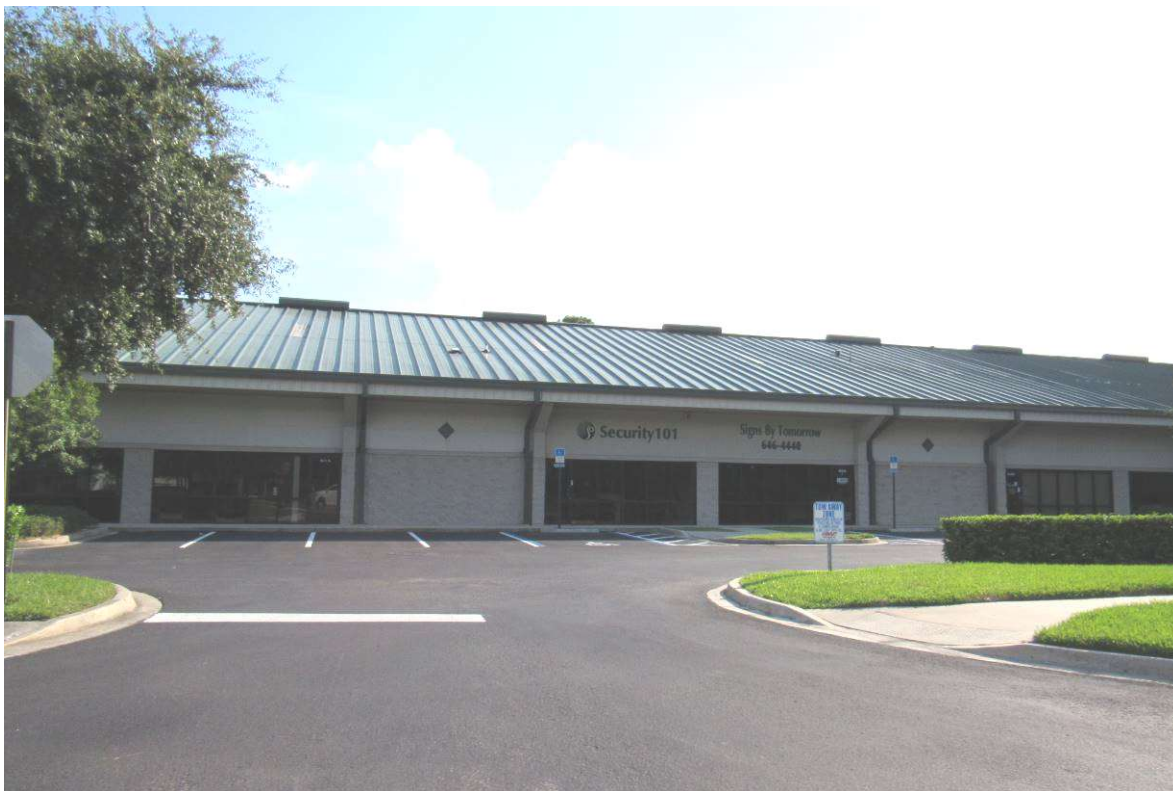
Adjacent office buildings
